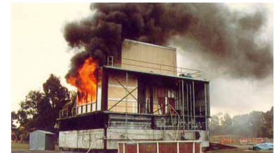
view of test structure showing fire in office above imposed little threat to the carpark below
